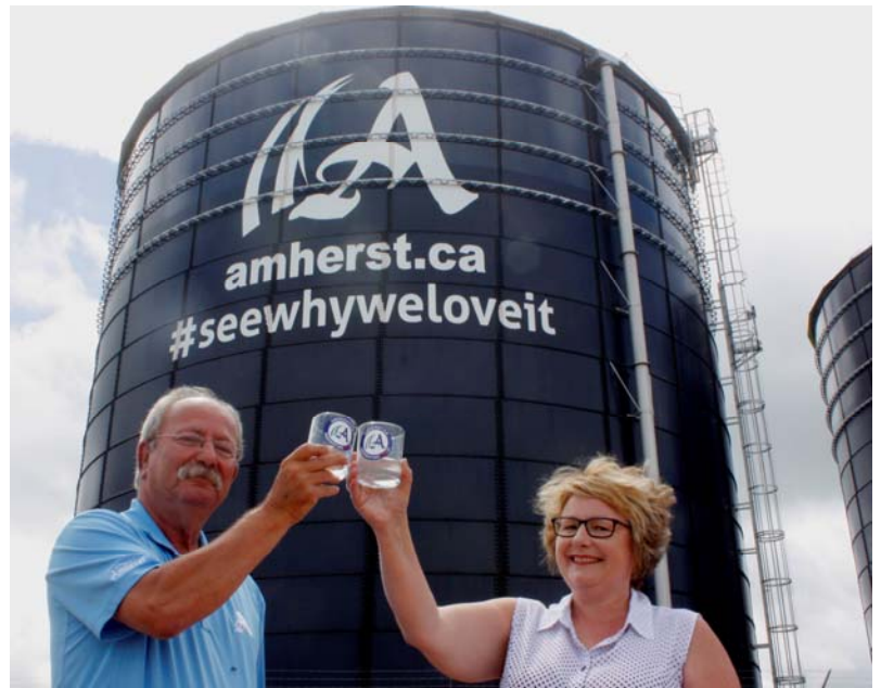
Mayor David Kogon and Deputy-Mayor Sheila Christie toast the commissioning of Amherst's new reservoir. The two tanks can hold 13 million litres of water. (Town of Amherst photo)
