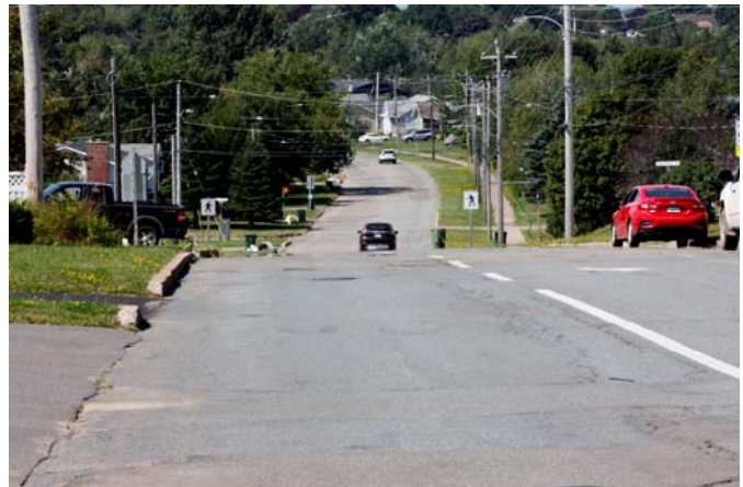
The Willow Street infrastructure renewal project is scheduled to begin on Sept. 12. (Town of Amherst photo)
