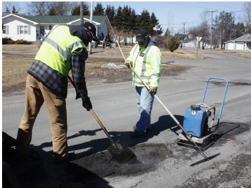
Public Works employees Lester Fromm and Dusty Collins repair potholes on Park Street. (Tom McCoag / Town of Amherst)
