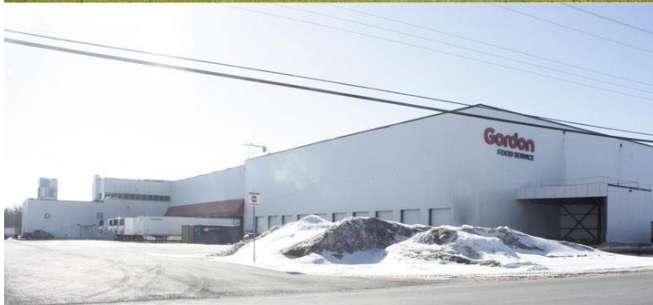
Work on the expansion of Gordon Food Service began last summer and is expected to be completed later this spring. (Tom McCoag / Town of Amherst)
