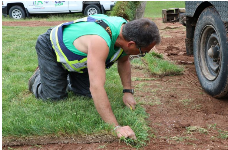
Chris Comeau trims some of the sod that was laid on the Robb 3 baseball field. The new sod helps to eliminate a lip between the infield and outfield. (Tom McCoag / Town of Amherst)
