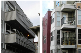
Figure 7. The balconies on the left offer more privacy and hide stored furniture better than those on the right.
