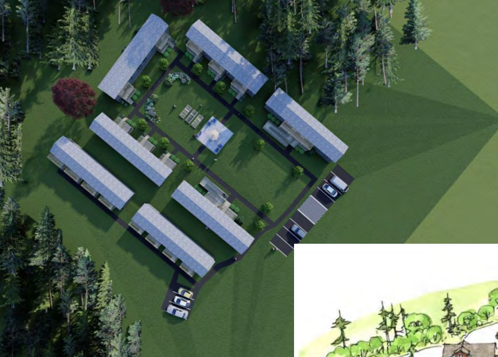
New Glasgow, NS Under Construction
