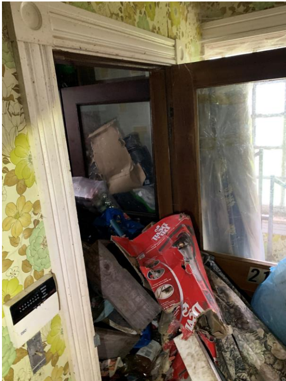
Main floor hoarding.
