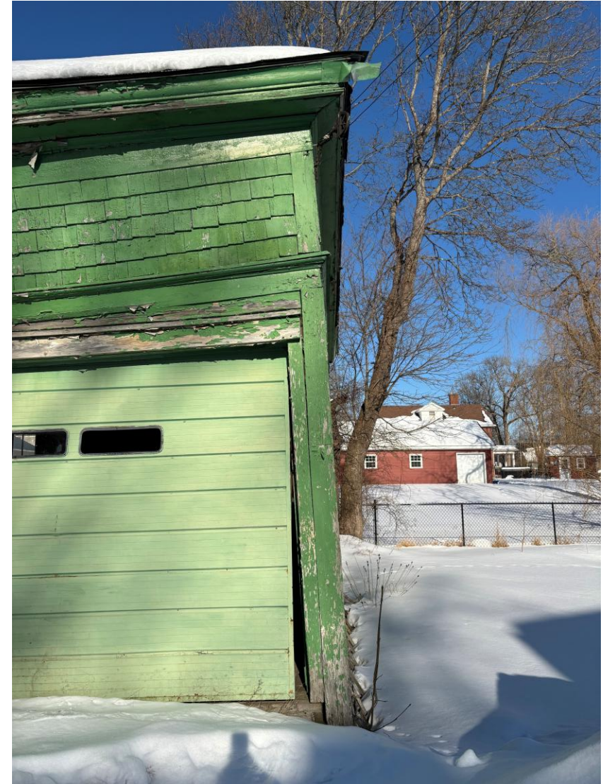
Exterior walls showing signs of structural fatigue; beginning to fall inward and twisting
