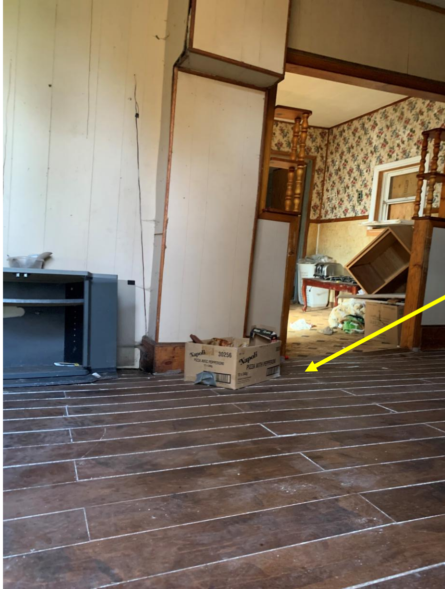
Significant bowing in floor
