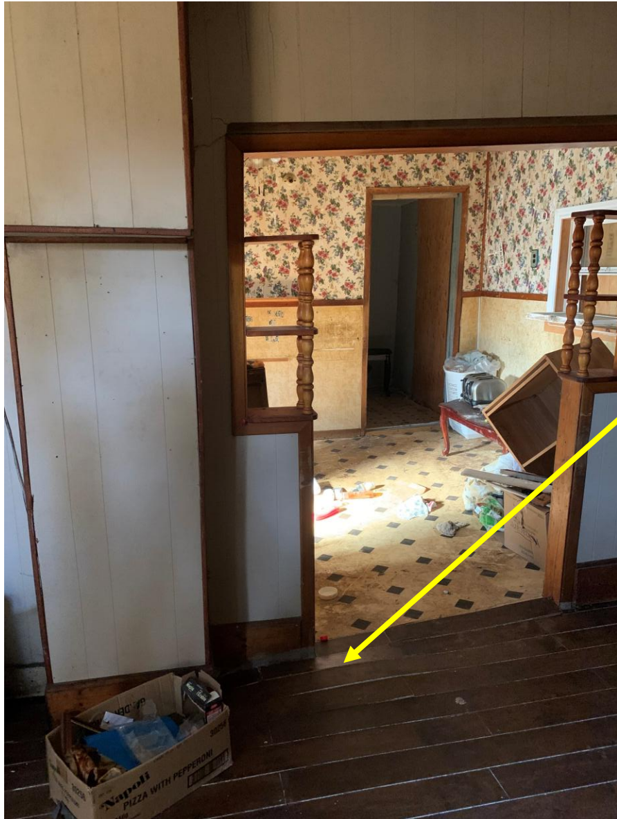
Significant bowing in floor
