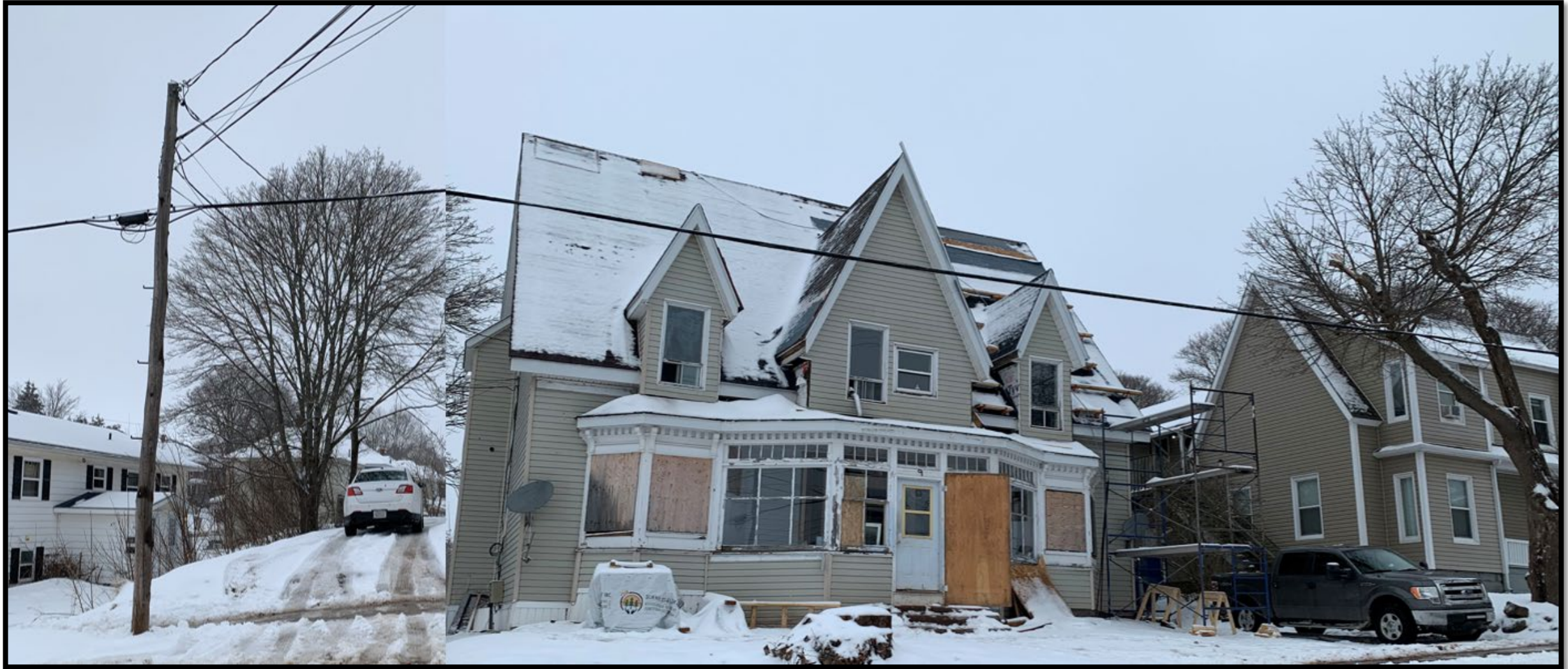
View of the subject property from North Adelaide Street
