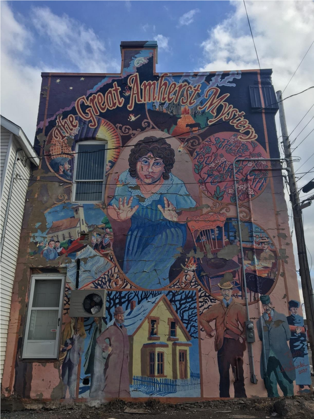
Located at the back of the building on the corner of LaPlanche & Victoria St. this mural was painted directly on the building by Susan Tooke & Richard Rudnicki in 2007. This mural has noticeable peeling in several areas.
