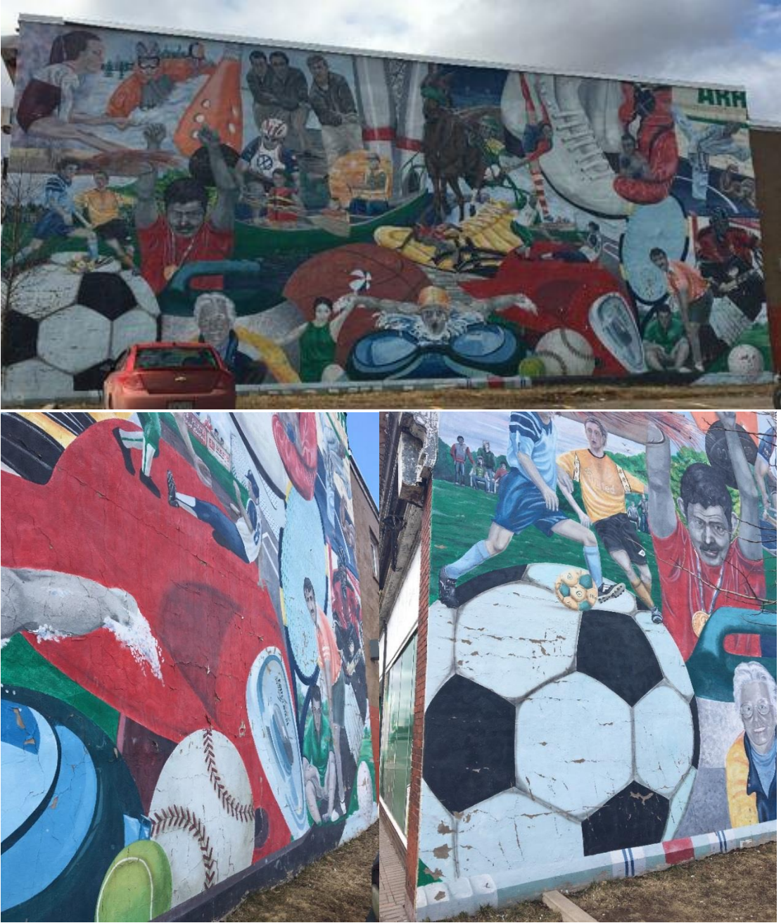
Located on the side of 50 Church St. painted in 2005 by Daren White this mural is beginning to peel in several areas. It is in fair condition.
