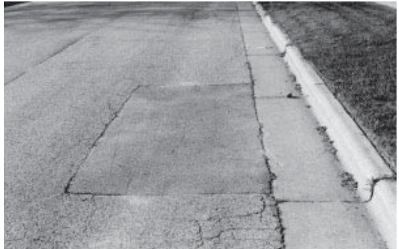
▼ Extensive block cracking. Blocks tight and sound. ◀ Slight rutting in wheel path.
