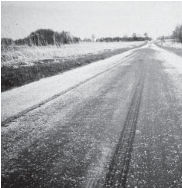
▼ Severe flushing.
