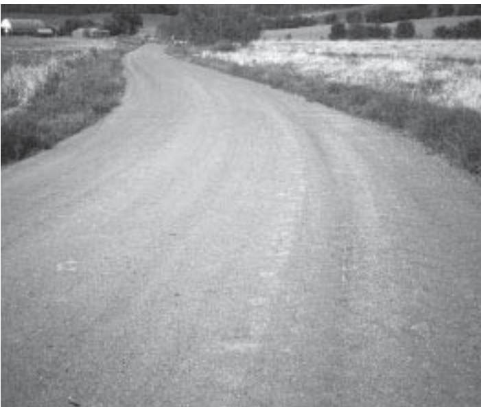
▲ New cold mix surface.
