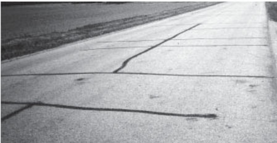
▼ Open crack, 1/2" wide; adjoining pavement sound.
