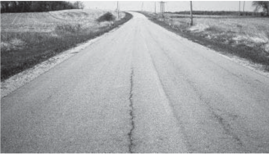
▼ Slight rutting; patch in good condition.
