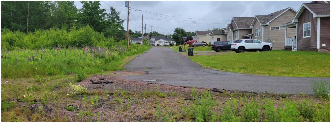
Moshier Street looking east to Walter Purdy Avenue at Gallagher Street
