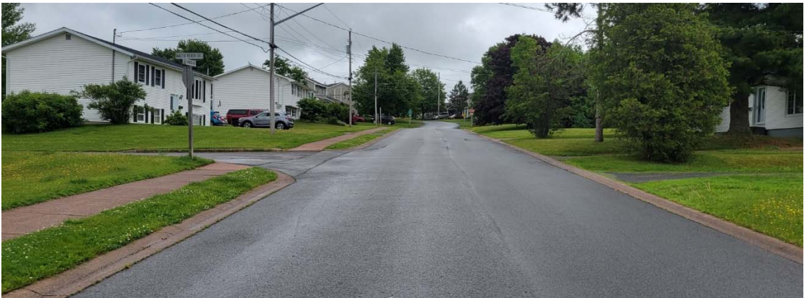
Donald Street at Walter Purdy Avenue looking east
