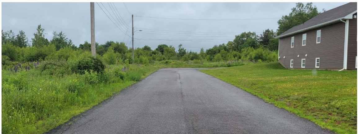
Existing northern end of Gallagher Street to be extended to Willow Street
