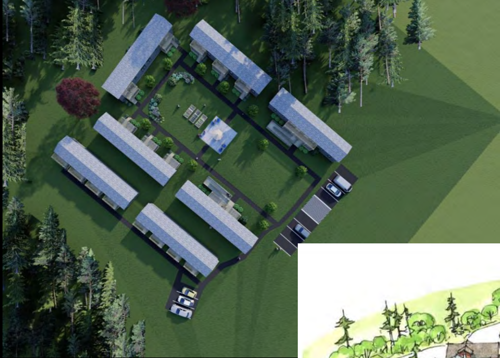
New Glasgow, NS Under Construction
